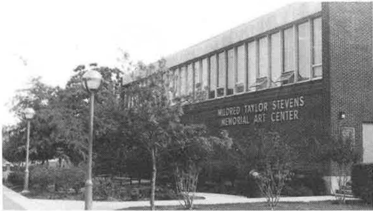
Stevens Art Gallery is slated to undergo a building addition beginning during the late fall. Professors' offices, the classrooms, and gallery will be relocated during the construction. Photo by Channing Bradford.
