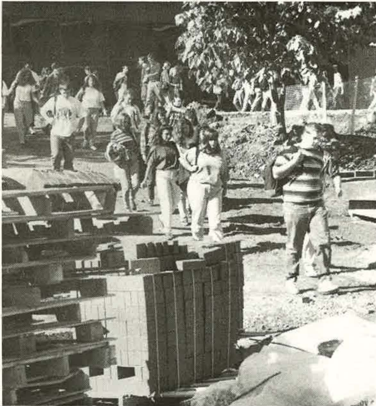
Watch your step. Students wind through the maze of construction in front of the Benson, anticipating the completion of the pedestrian mall. Photo by Nathan Ironside.
