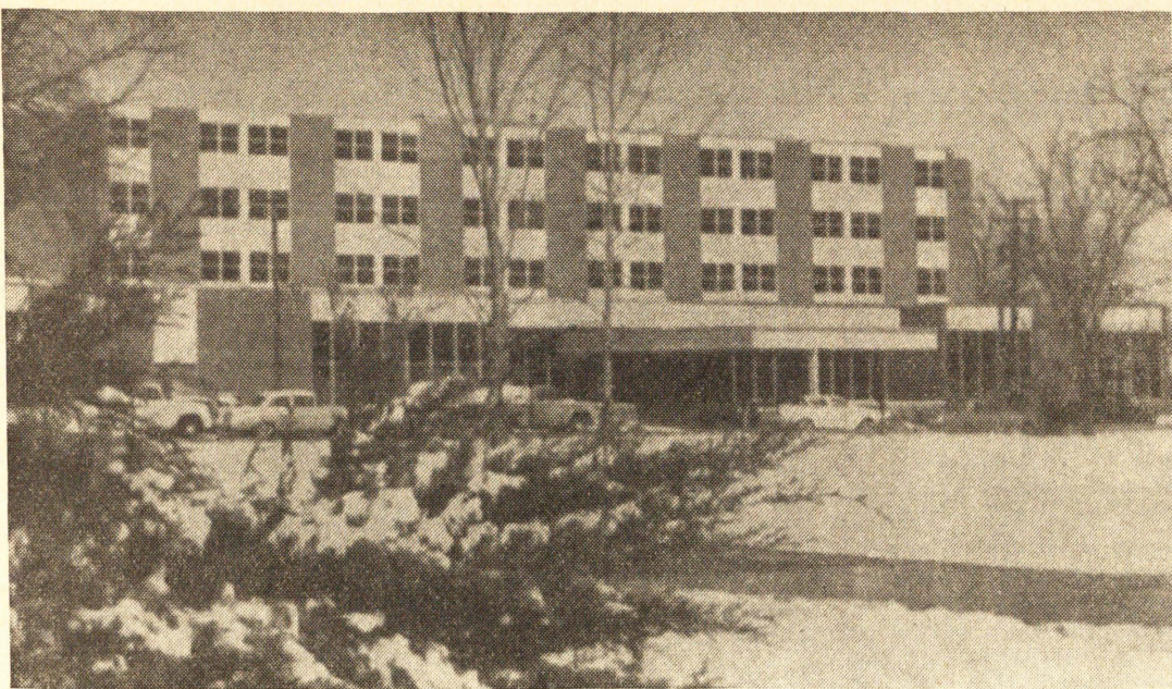
A TWO-INCH BLANKET of snow which fell last week makes a beautiful setting for the almost-completed American Heritage and Alumni Center which will be opened later this spring.
