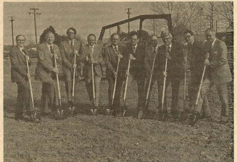
Manning the shovels during the March 20 groundbreaking for the J. E. Mabee Business Center are (left to right) Floyd Daniel, Clifton Ganus, David Burks, Del Belden, Jack Wiseman, Lott Tucker, James Cone, Dwane Treat, J. E. Pryor and Randall Yearwood.
