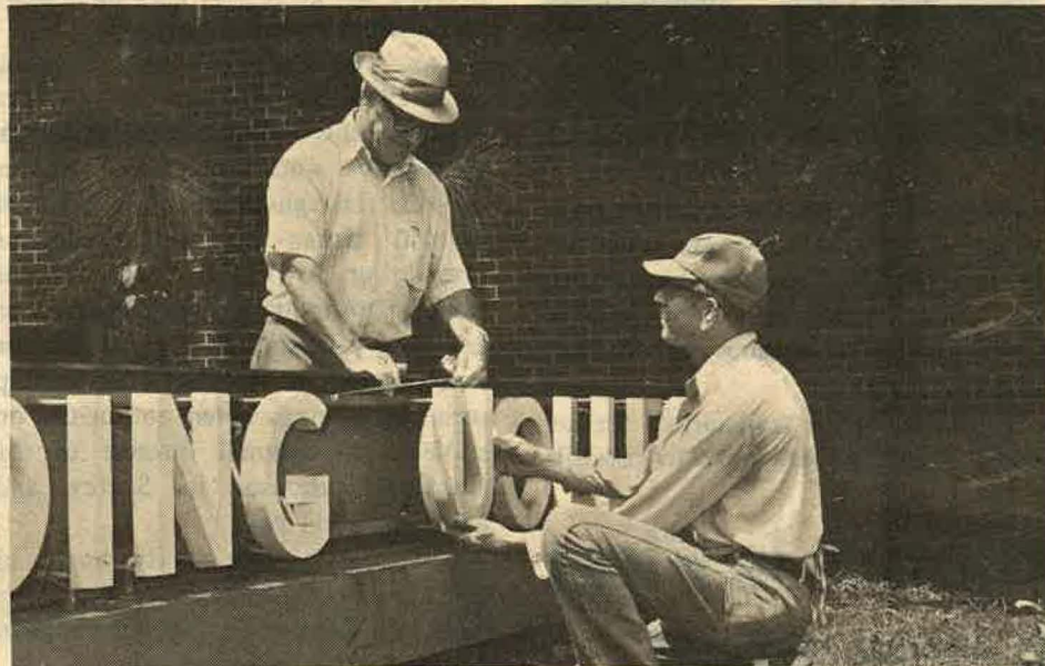
Preparing to make one of several changes for the new University name, construction superintendent W. T. "Shorty" Pearson and assistant Tom James measure for new lettering on the American Heritage sign.
