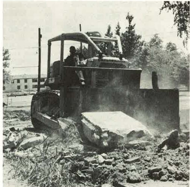
Clearing Ground for a New Women's Dormitory
