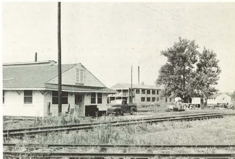
Three moved buildings make strange neighbors across tracks.
