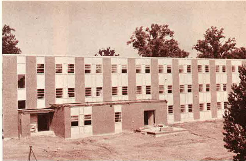
One wing of new men's dormitory will be ready soon.
