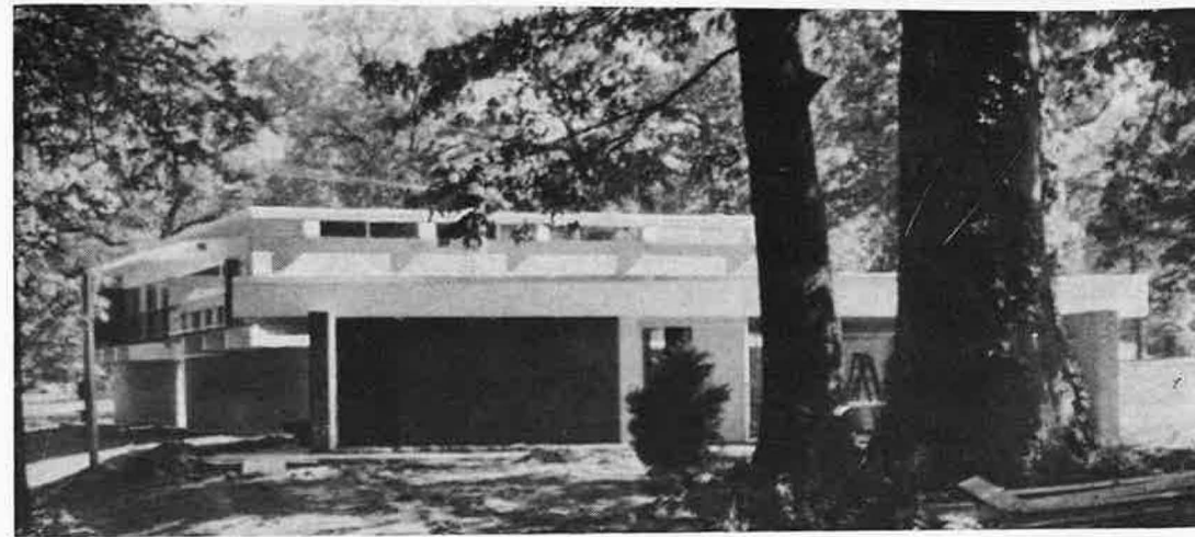
The New 20-Room Dormitory for the Graduate School of Bible and Religion in Memphis
