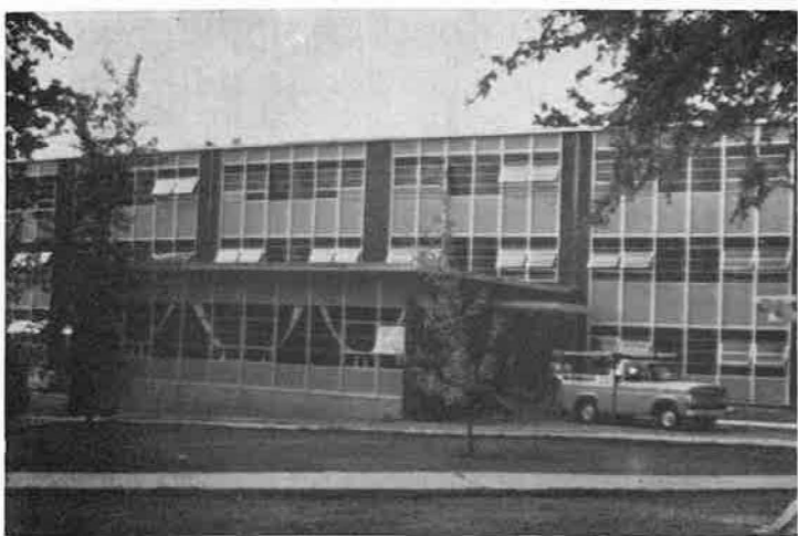
This is how the new dormitory looks from the court between Cathcart and Pattie Cobb Halls. The new-style window units add to its symmetry.
