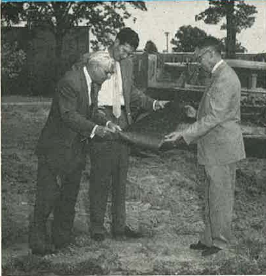
Dr. Benson explains plans for the new Bible Building to professors James D. Bales and Conard Hays of the Bible Department while grading equipment is at work preparing the foundation. Completion is estimated for June, 1960.
