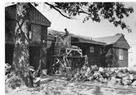
Dean Mattox finishing up his chimney of Arkansas field stone.
