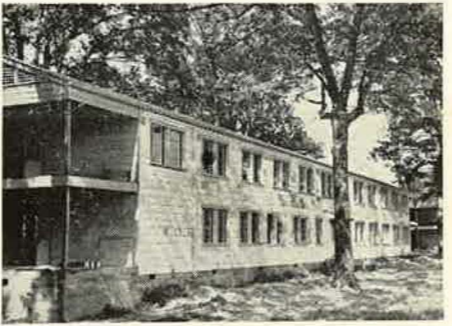
One of two men's dormitories nearing completion.
