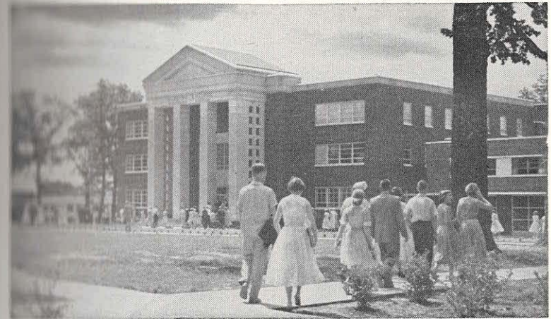
The Administration-Auditorium Building is center of activity.
