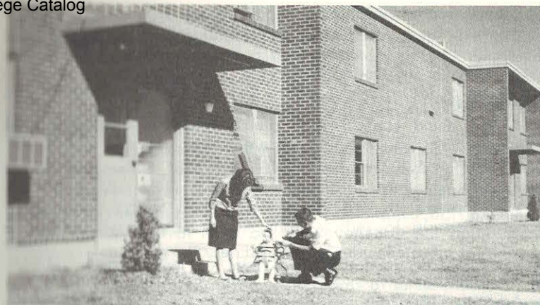
A Section of the 60-unit Married Students Apartments.
