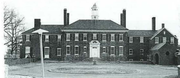
The Old Mansion is the main structure on the campus of the Graduate School of Religion in Memphis, Tenn.
