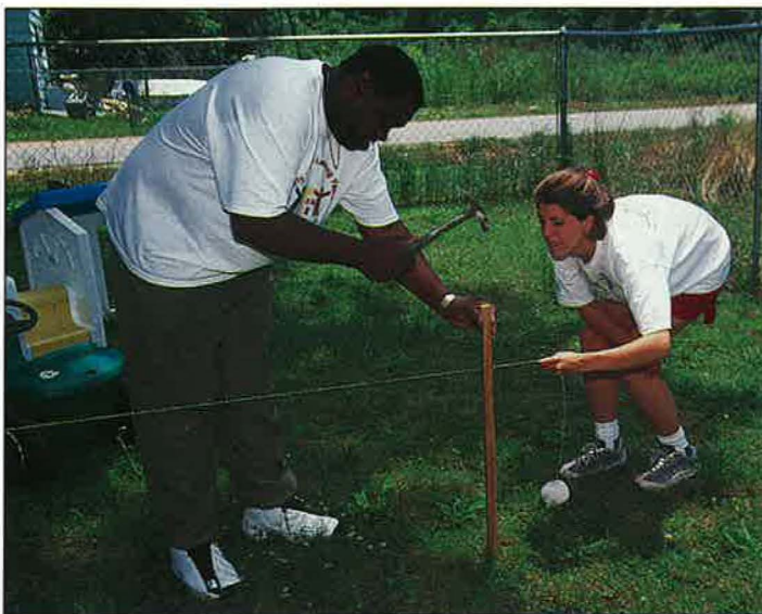
Stake Out. Senior Caroline Craig holds the rope-line straight for David Green. The Greens plan to build an addition to their Center to accommodate the many children on the waiting list.
