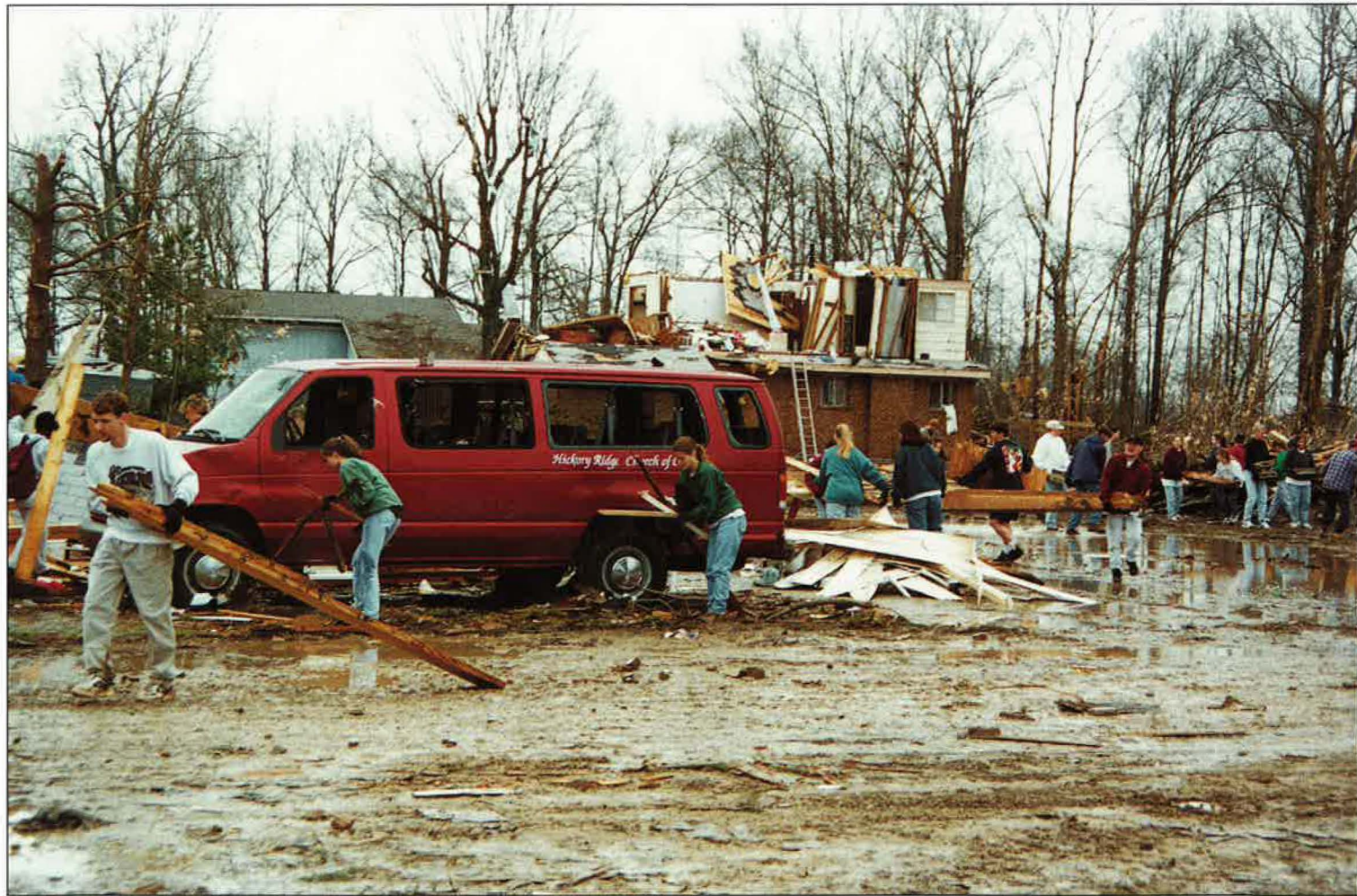
Picking Up the Pieces. After tornados ravaged Arkansas in March, students clean up debris from the Hickory Ridge Church of Christ, which was totally destroyed.
