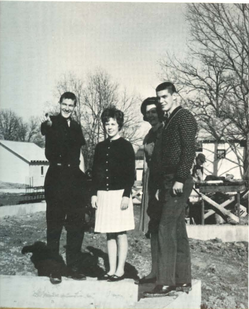
DREAMING of the completion of the newest construction on campus, seniors point out various foundations of the alumni building with pride.
