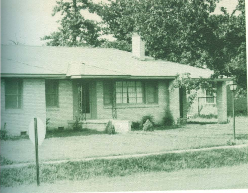
THE HOME MANAGEMENT HOUSE —named Echo Haven, offers valuable training in various phases of household management.
