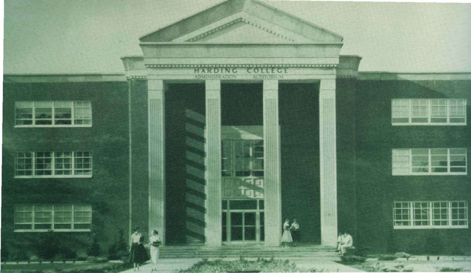
THE ADMINISTRATION-AUDITORIUM BUILDING —contains administrative and faculty offices, Little Theatre, recording studios, classrooms, and the main auditorium with a seating capacity of 1,350, all of which are air-conditioned.
