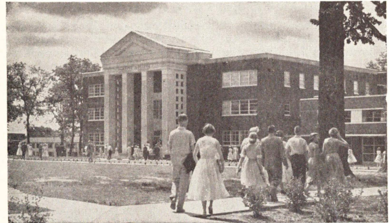
The Administration-Auditorium Building is center of activity.
