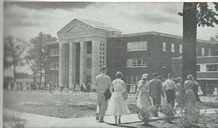
The Administration-Auditorium Building is center of activity.
